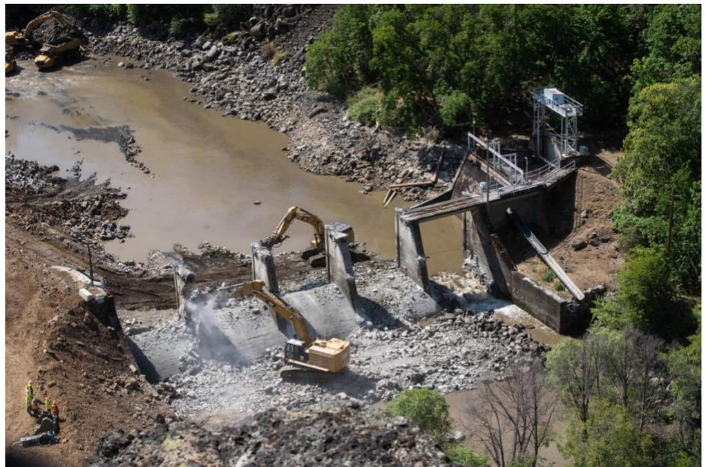
Crews placed around 10 feet of rock on either side of the dam in order to reach the gates and bays for deconstruction. Much of the Copco No. 2 infrastructure remains in place below this rock surface. Deconstruction of this dam will continue through the summer, with final decommissioning and complete removal occurring sometime in September.
